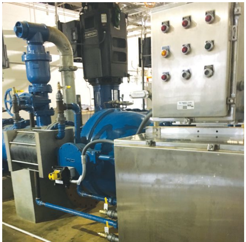
Image 1. Smart ball valve pump control system (Images courtesy of Val-Matic Valve & Mfg. Corp.)
