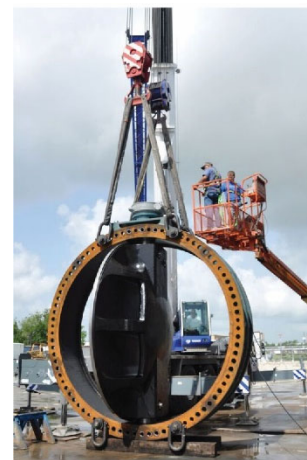
FIGURE 5. Use of Swivel Rings to lift a 144-inch Butterfly (Courtesy of United Valve)
