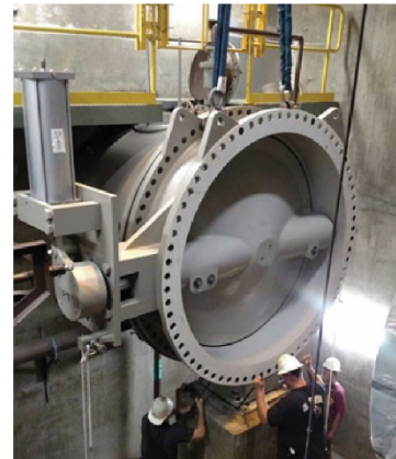
FIGURE 1. Installation of 90-inch Butterfly Valve
