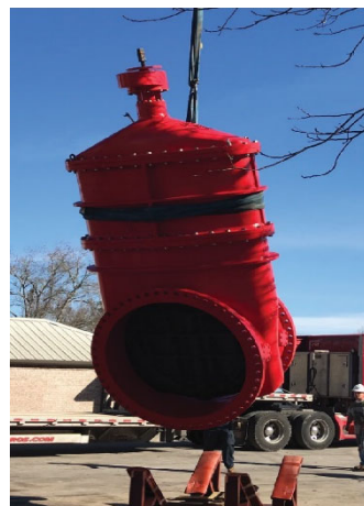
FIGURE 4. Hoisting a 60-inch Gate Valve (Courtesy of J&S Valve)
