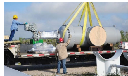
FIGURE 2. Unloading of a 36" Pipeline Valve (Courtesy of United Valve)
