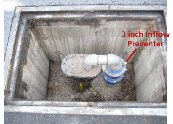
FIGURE 6. Air Valve Vault, Foster City, CA
