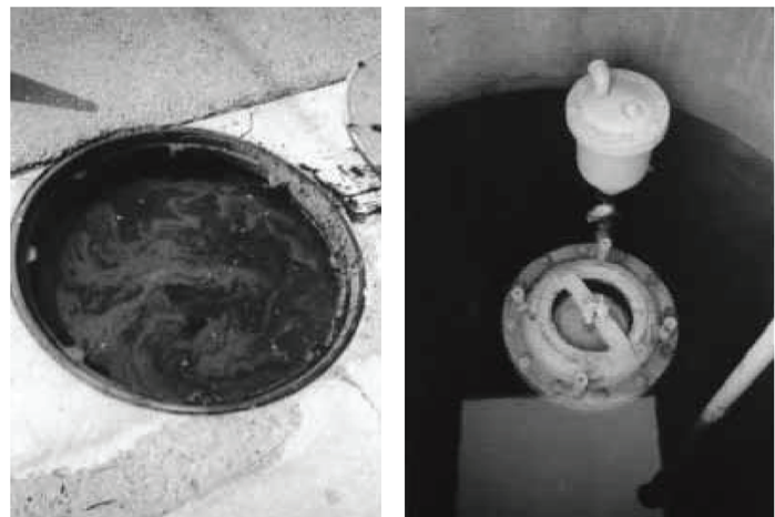
FIGURE 1. Submerged Air Valve Vault (LeChevallier)
