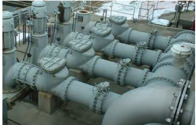
FIGURE 1. Typical Pumping System with Swing Check Valves
