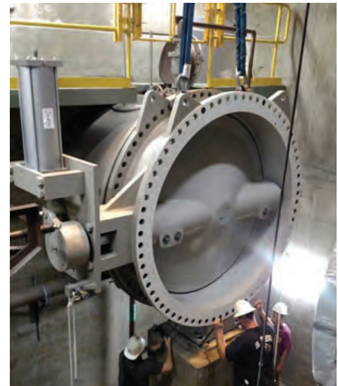
FIGURE 1. Installation of 90-inch Butterfly Valve
