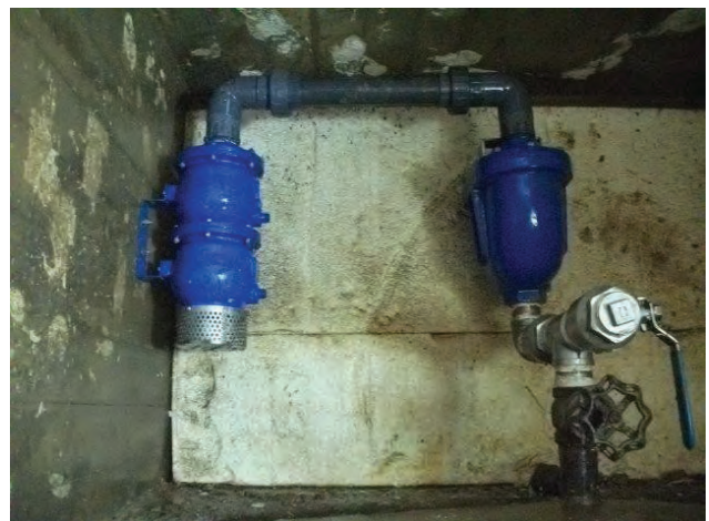
FIGURE 4. Typical ASSE 1063 Inflow Preventer Installation
