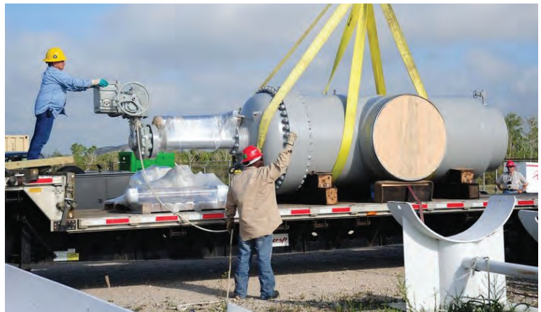
FIGURE 2. Unloading of a 36" Pipeline Valve (Courtesy of United Valve)
