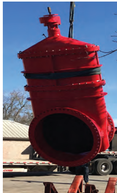
FIGURE 4. Hoisting a 60-inch Gate Valve (Courtesy of J&S Valve)
