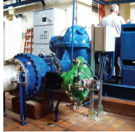
FIGURE 1. Pump Control Ball Valves in Ohio, USA
