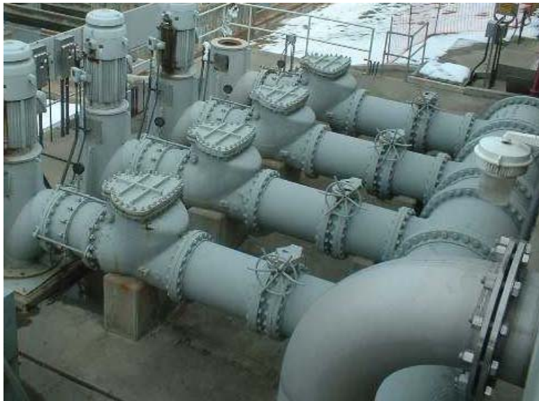
FIGURE 1. Typical Pumping System with Swing Check Valves
