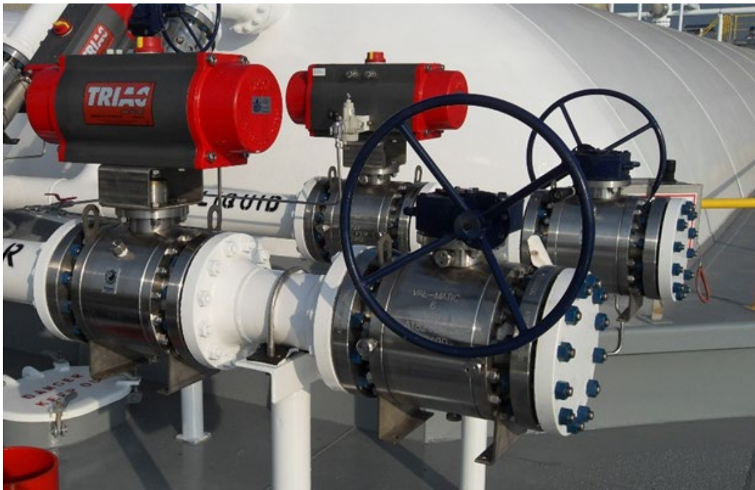
Figure 1. Trunnion-Mounted Ball Valves (Courtesy of Val-Matic Valve)
