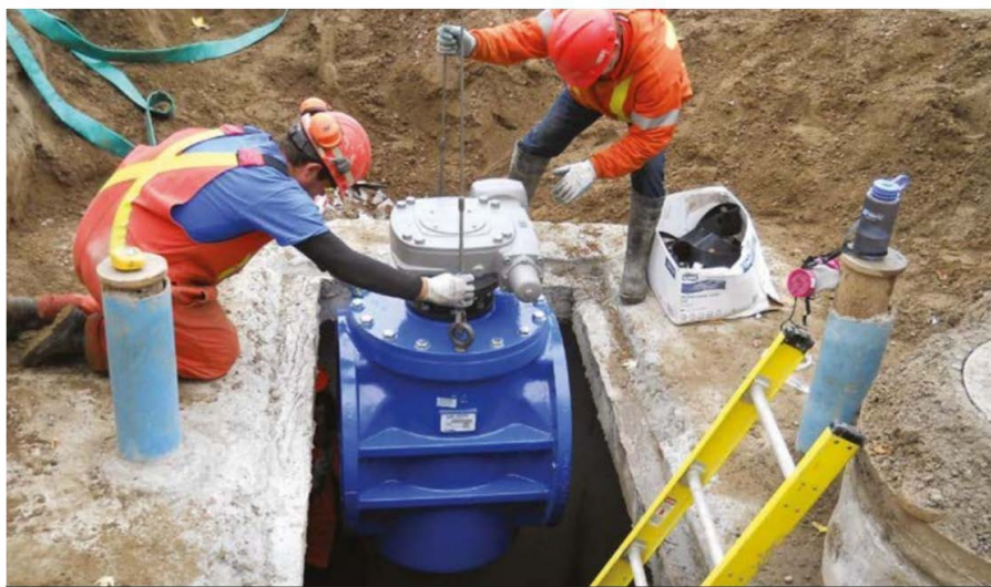
Figure 1. Installation of 24-inch plug valve in a vault in Collingwood, Ontario
