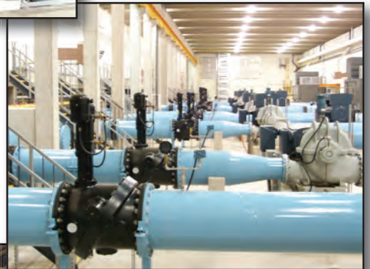
Tilted Disc® Check Valve with Top Mounted Oil Dashpot.
