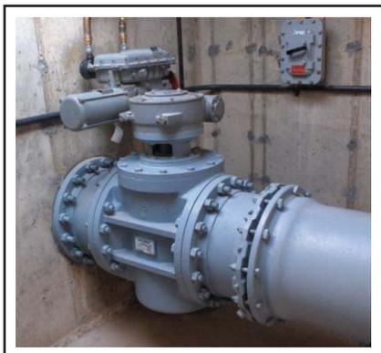
Cam-Centric® Plug Valve with motor actuator
