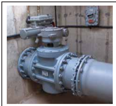
Cam-Centric® Plug Valve with motor actuator
