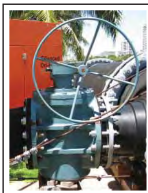
Cam-Centric® Plug Valve with worm gear actuator
