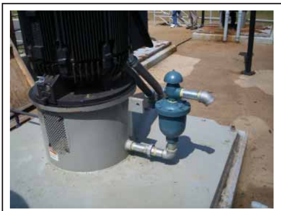
Air/Vacuum Valve with Dual Port Throttling Device
