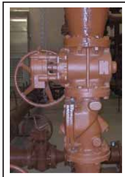
Cam-Centric® Plug Valve with Val-Matic Swing-Flex®
