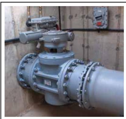
Cam-Centric® Plug Valve with motor actuator
