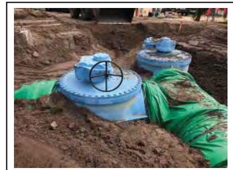
Cam-Centric® Plug Valve with worm gear actuator
