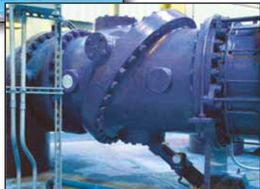
Tilted Disc® Check Valve with Bottom Mounted Oil Dashpot.
