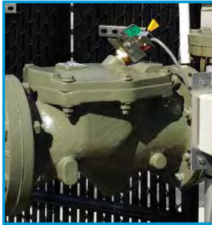
Swing-Flex® Check Valve with Limit Switch
