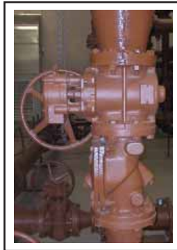
Cam-Centric® Plug Valve with Val-Matic Swing-Flex®
