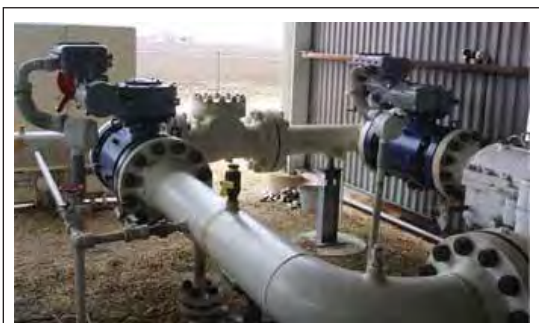
Crude Oil Pumping Station Pig Launcher/Receiver
