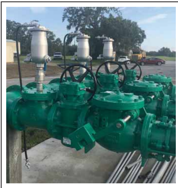
Single Body Wastewater Combination Air Valve
