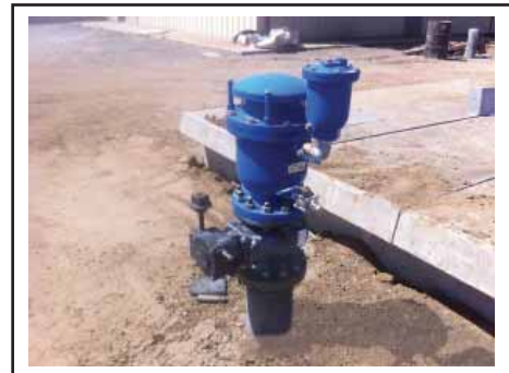
Cam-Centric® Plug Valve with Val-Matic dual body combination Air Valve
