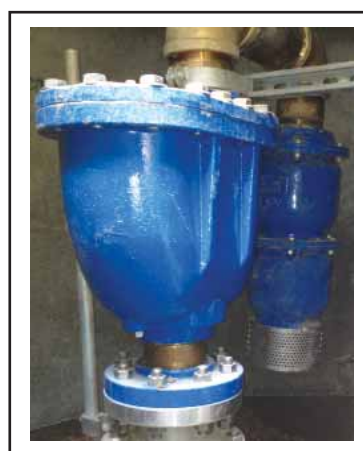
Single Body Combination Air Valve with FloodSafe® Inflow Preventer
