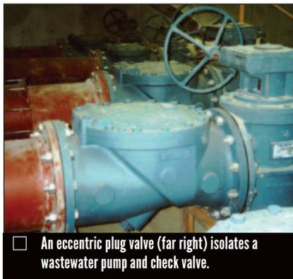
□ An eccentric plug valve (far right) isolates a wastewater pump and check valve.
