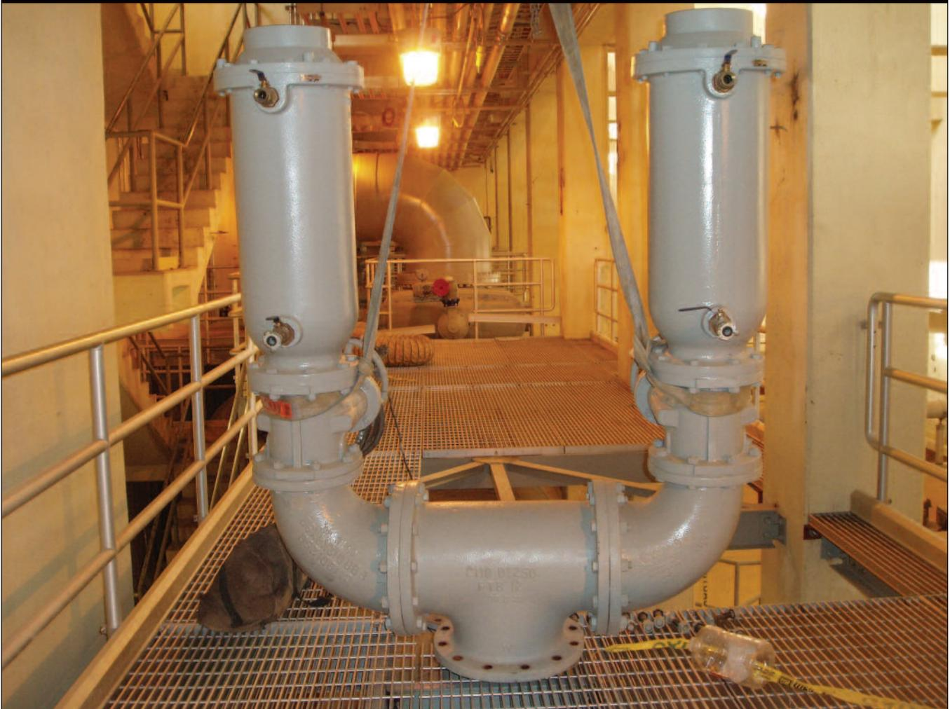
accordance with Manufacturers Standardization Society (MSS) SP-108 or AWWA C517. The seat and plug face of an eccentric plug valve is located offset from the valve shaft and port so that, as the plug is rotated out of the seat, it is pulled away rather than scraping against that seat. This eccentric action prevents wear in abrasive service. Moreover, if wear does occur, the actuator can be adjusted, further closing the plug to provide new seating surface and a tight seal.
