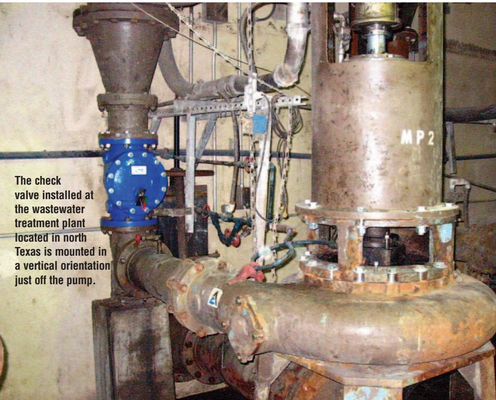
The check valve installed at the wastewater treatment plant located in north Texas is mounted in a vertical orientation just off the pump.
