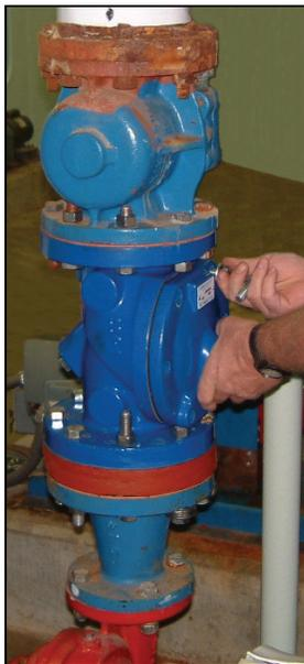
In the installation shown in the photo, a four-inch Surgebuster is being installed in an existing high-dynamic auxiliary water system to resolve serious slamming issues. The check valve is mounted in a vertical line upstream of a 70-psig hydro-pneumatic tank which caused swing check and dual disc check valves to slam. A Surgebuster was installed and monitored with a data acquisition system. The results found the Surgebuster closed in about 1/8 of a second with near silent closure.
