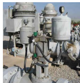
Leaking Dashpot
