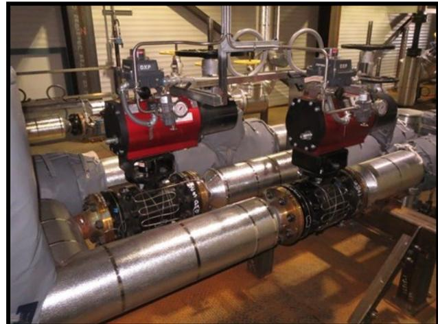
Figure 4. New well pad module with 4" ANSI 600 QuadroSphere® Ball Valves at Suncor Firebag SAGD Facility
