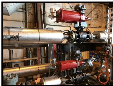
Figure 5. 2" and 3" ANSI 600 QuadroSphere® Ball Valves with Rotork Actuators and Fisher DVC position transmitters at Suncor Firebag SAGD facility.
