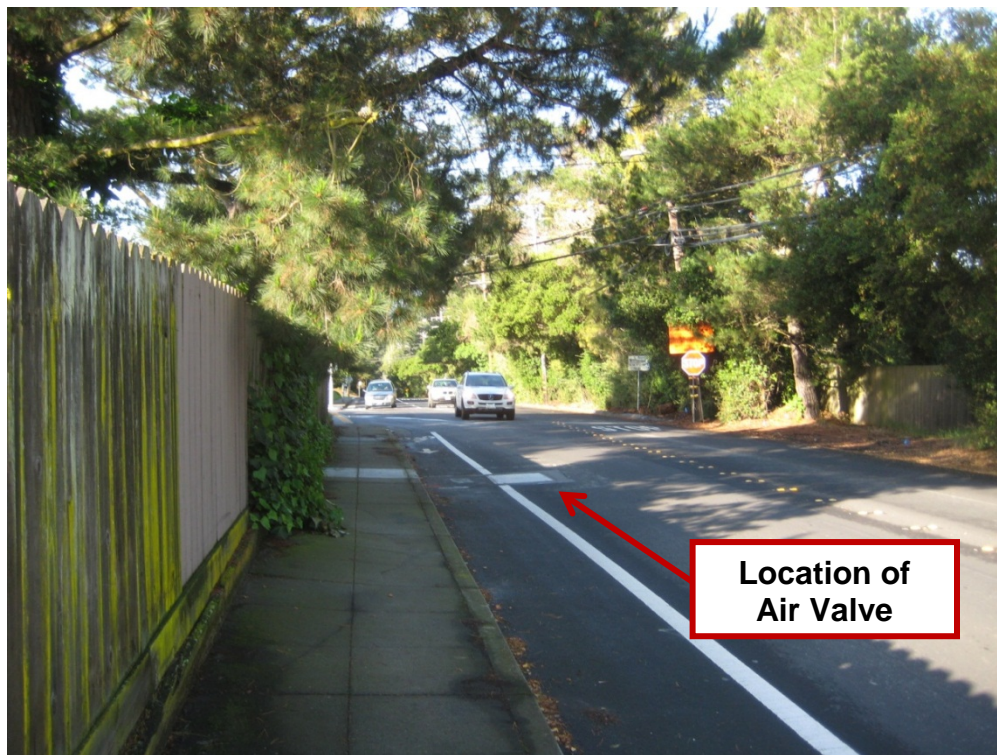
FIGURE 5. Water Pipeline in Foster City, CA
