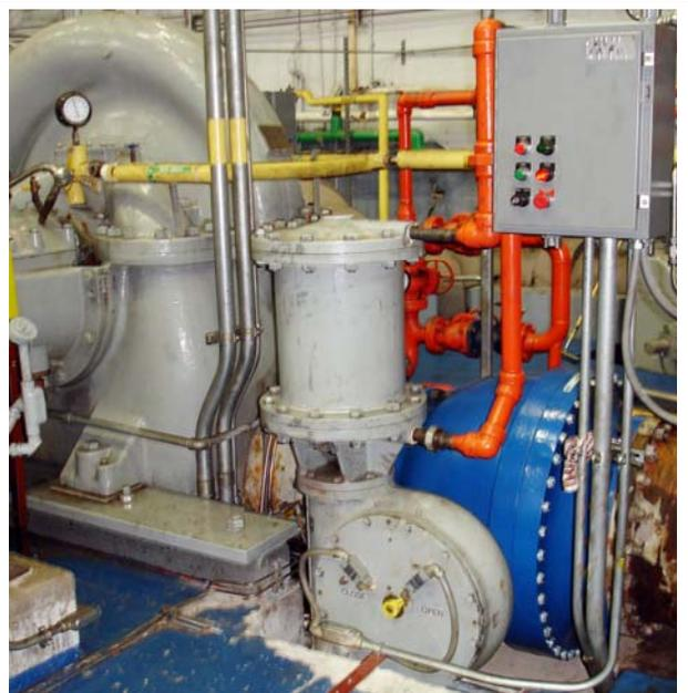
**Ener•G® Ball Valve installed at Roseland Pumping Station, Chicago, IL**
