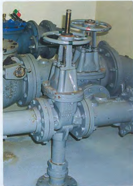
The check valves in question at the Mt. Horeb, Wis., Wastewater Treatment Plant were allowing sewage to build up on top of the disc, restricting the effectiveness of the valve, causing it to slam.
