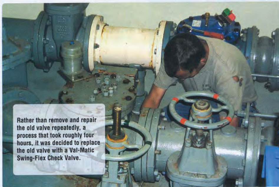
The check valves in question at the Mt. Horeb, Wis., Wastewater Treatment Plant were allowing sewage to build up on top of the disc, restricting the effectiveness of the valve, causing it to slam.
