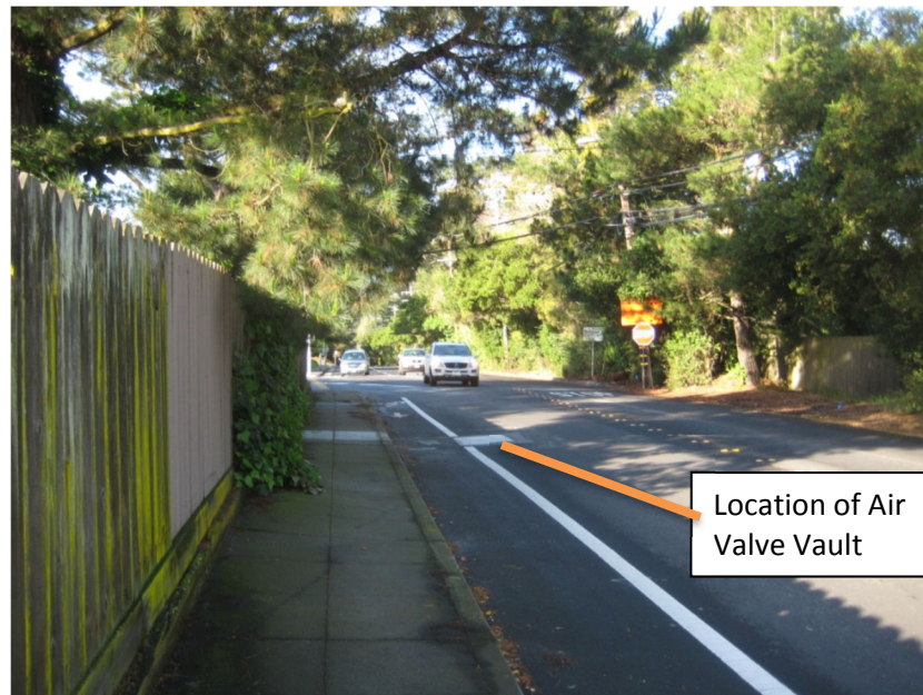
FIGURE 5. Water Pipeline in Foster City, CA
