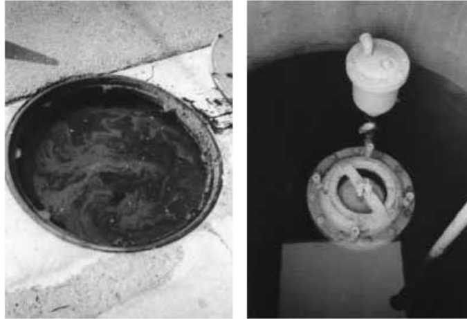
FIGURE 1. Submerged Air Valve Vault (LeChevallier)
