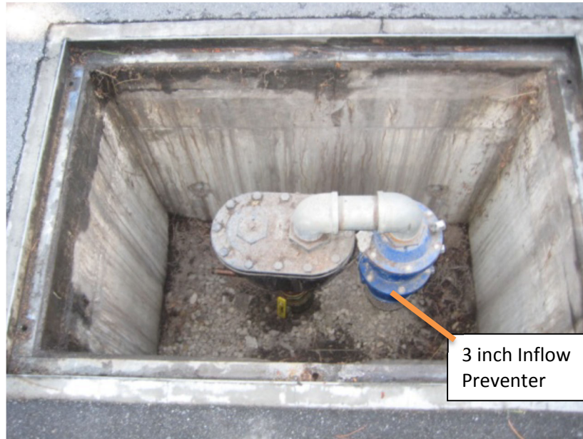
FIGURE 6. Air Valve Vault, Foster City, CA
