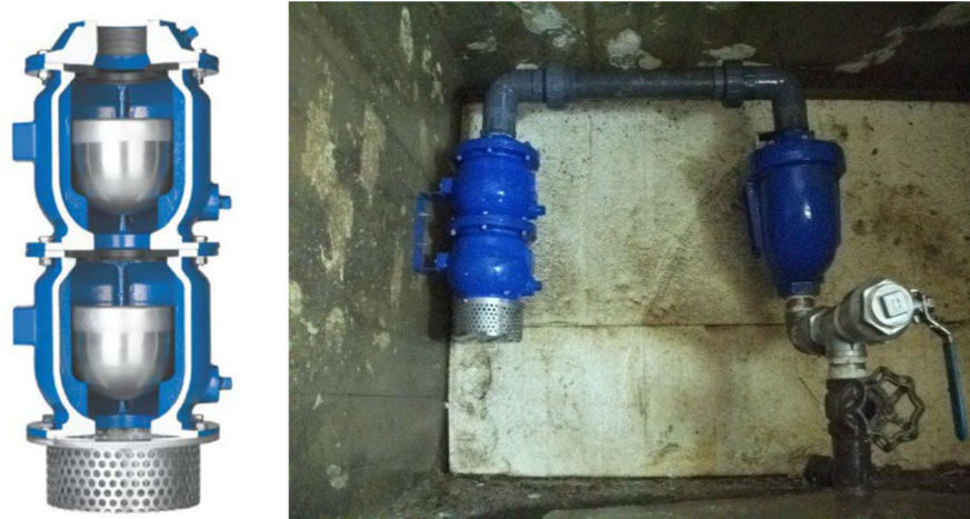
FIGURE 4. Typical ASSE 1063 Inflow Preventer Installation
