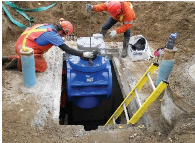
FIGURE 1. Installation of 24 in. plug valve in a vault in Collingwood, Ontario
